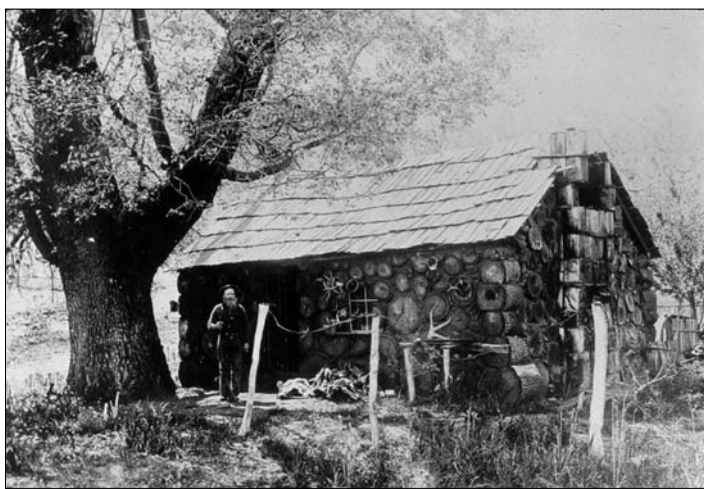
Shepherd's Cabin Made of Piled Short Oak Logs by A.O. Carpenter
